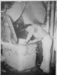
The Chief Engineer of the Kosmos III inspects one of the tanks in the hold. Before loading they are painted with a washable coating which can be holed down when the fuel oil is consumed. Then the valuable whale oil is placed in the empty, clean tanks. In addition to fuel oil, 19,112 barrels of diesel were loaded.
